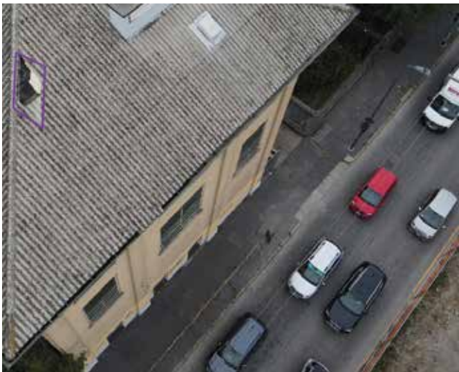
Above , Aerial inspection and thermography using drones for the automatic detection of anomalies in photovoltaic systems. Below , Verification of the maintenance status of building roofs through aerial inspection with drones for the detection and automatic classification of anomalies.
